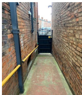
2. Turn left, go up the ramp to the fire exit gate.
