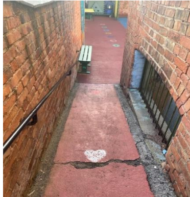
2. Turn right down the ramp
